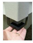
Start one leg of the Kritter-Cap<sup>TM</sup> into the corner post fold. Insert the other leg and push the Kritter-Cap<sup>TM</sup> up to the top of the foundation. If possible, use a small mirror to see that the Kritter-Cap<sup>TM</sup> is closing the gap.
